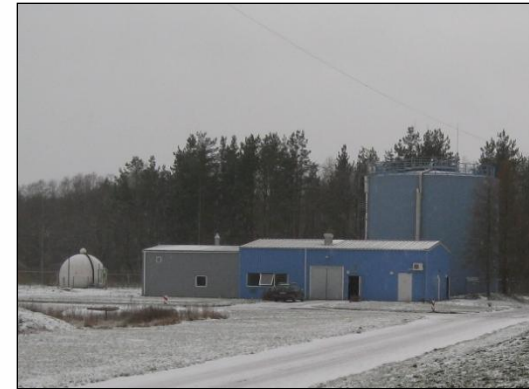
Photo 2. Narva Wastewater Treatment Plant 2
