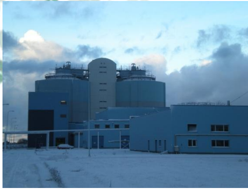
Photo 1. Tallinn Wastewater Treatment Plant 1
